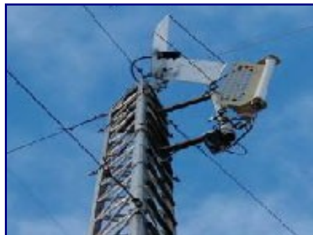
Figure 2: Solectek Antenna installed in Mérida, Venezuela, 1997 as part of RETIEM, (Merida State Teleinformatic Network) with links of up to 40 km.
